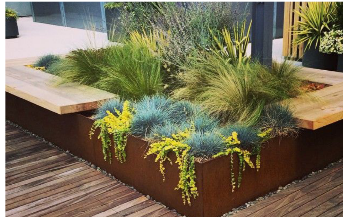
Roof deck planter, with timber decking terrace
