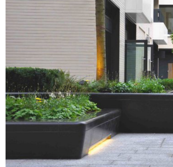
Lighting within raised planters
