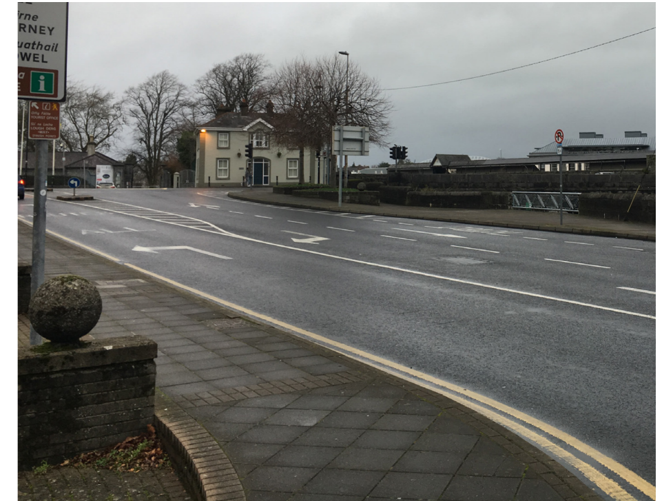
Pavements to be widened along Bank Place
