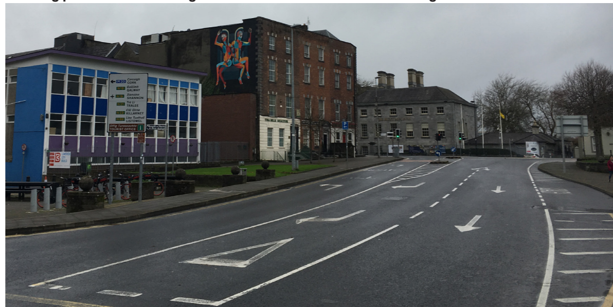
Existing wide carriage way on Bank Pl quayside
