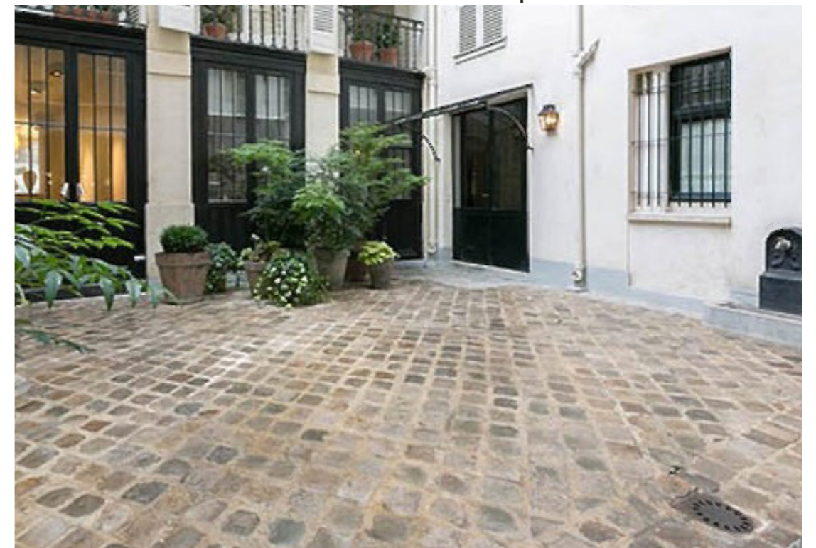
Granite sett paving
